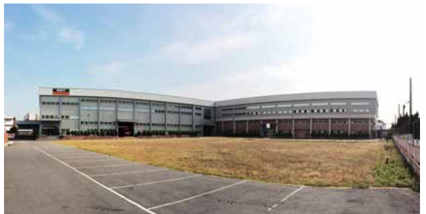
▲RST's new 11,000 m2 plant in Taichung.
